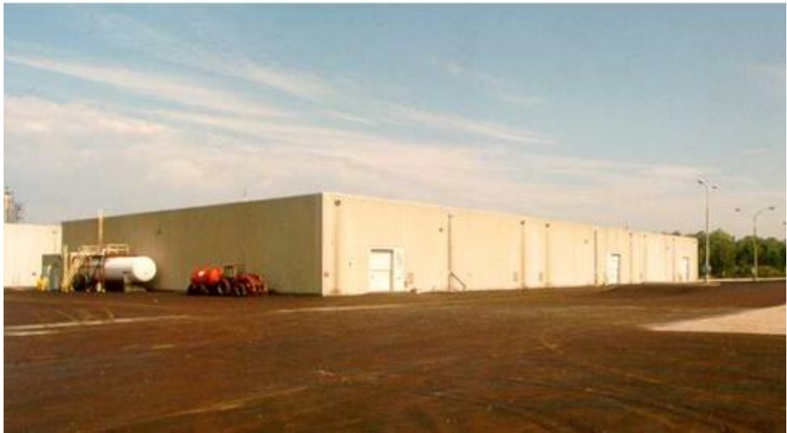
Figure 8: Low Level Storage Building
