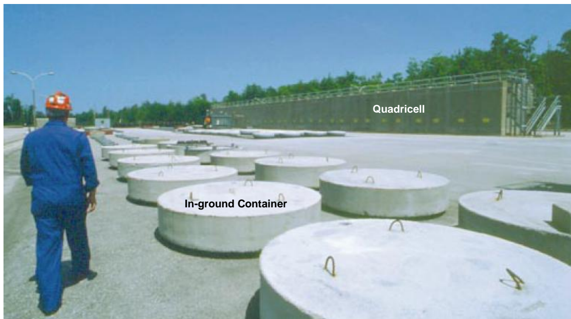
Figure 13: In-ground Containers (foreground) and Quadricells (background)
